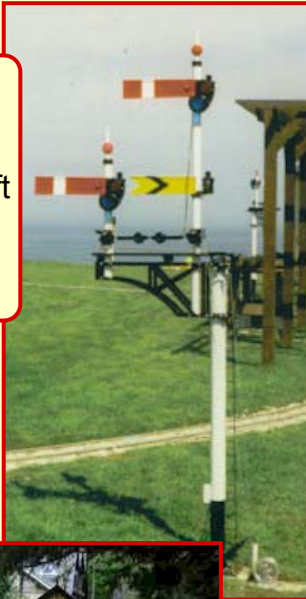
GWR lower quadrant right hand bracket, 1 doll with a 4ft home arm
